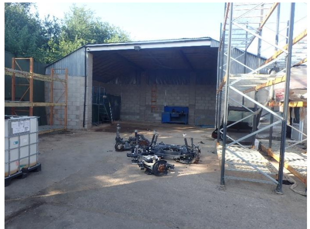
Open Sided Storage
